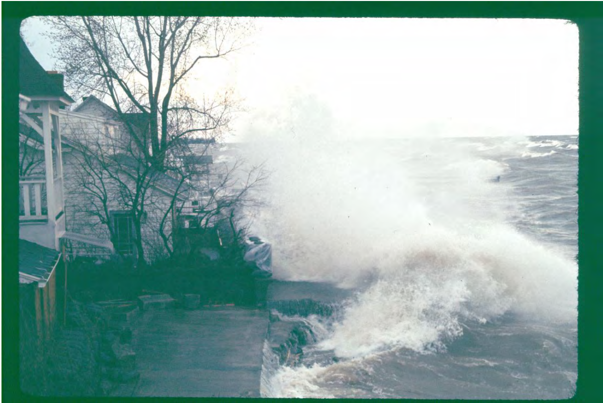
Figure D.3.1-7: Wave Overtopping on the coast of Lake Ontario for a 1973 Storm, Edgemere Drive, Monroe County, NY. Photo Courtesy of Dr. Martin
