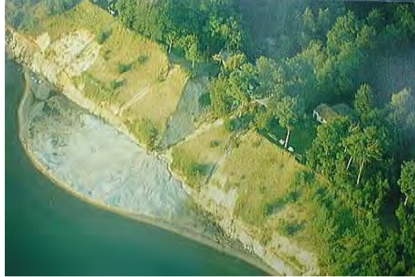
Figure D.3.7-7: Massive Slope Failure, St. Glenn Shores, Michigan
