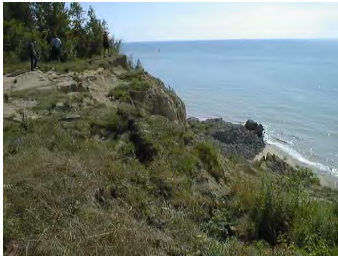
Figure D.3.7-9: Rotational Slope Failure in 1998, 107 th Street Allegan County, Michigan
