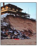
The two most damaging aspects of coastal flooding for coastal buildings are erosion and scour.
