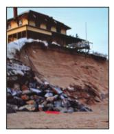
The two most damaging aspects of coastal flooding for coastal buildings are erosion and scour.
