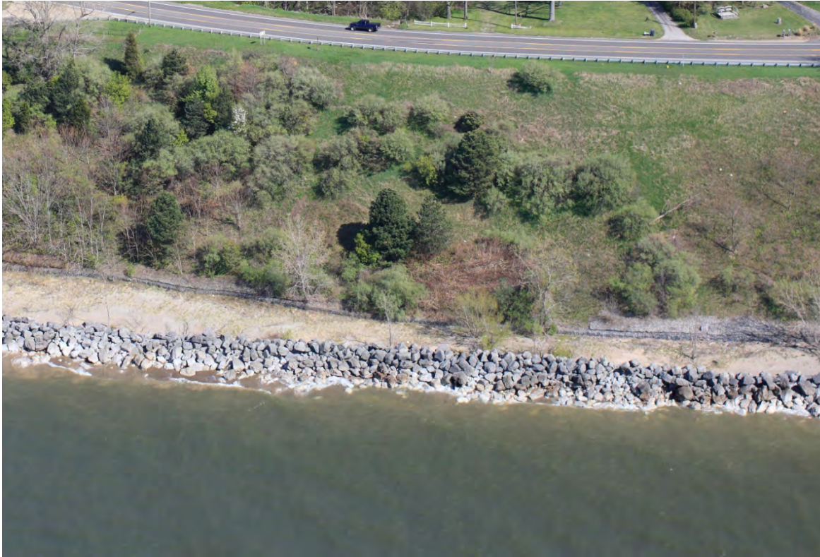
Figure 36: Stone Revetment along South Lakeshore Drive Oblique Photo
