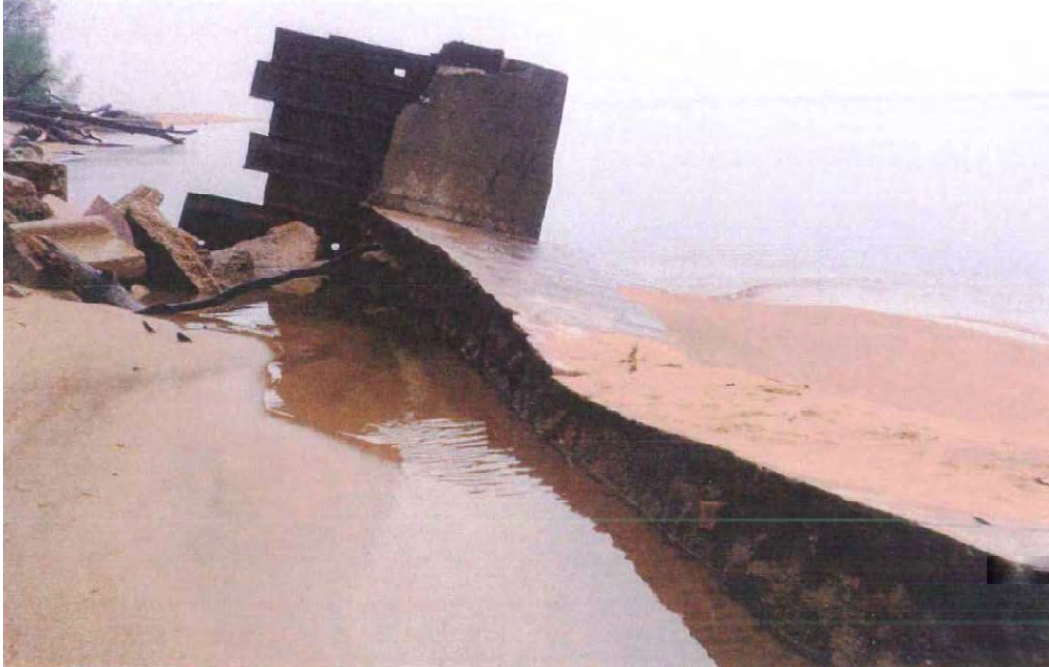
Figure 32: USACE CEM Photo, “A toppled concrete seawall along the Lake Michigan coast of Berrien County. Failure probably resulted from undermining of the underlying glacial till foundation, April 1991.”
