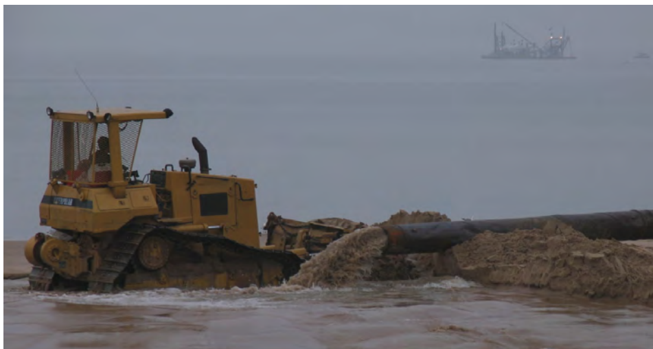
Figure 15: 2012 photo of beach nourishment south of Park Street showing the dredge in background
