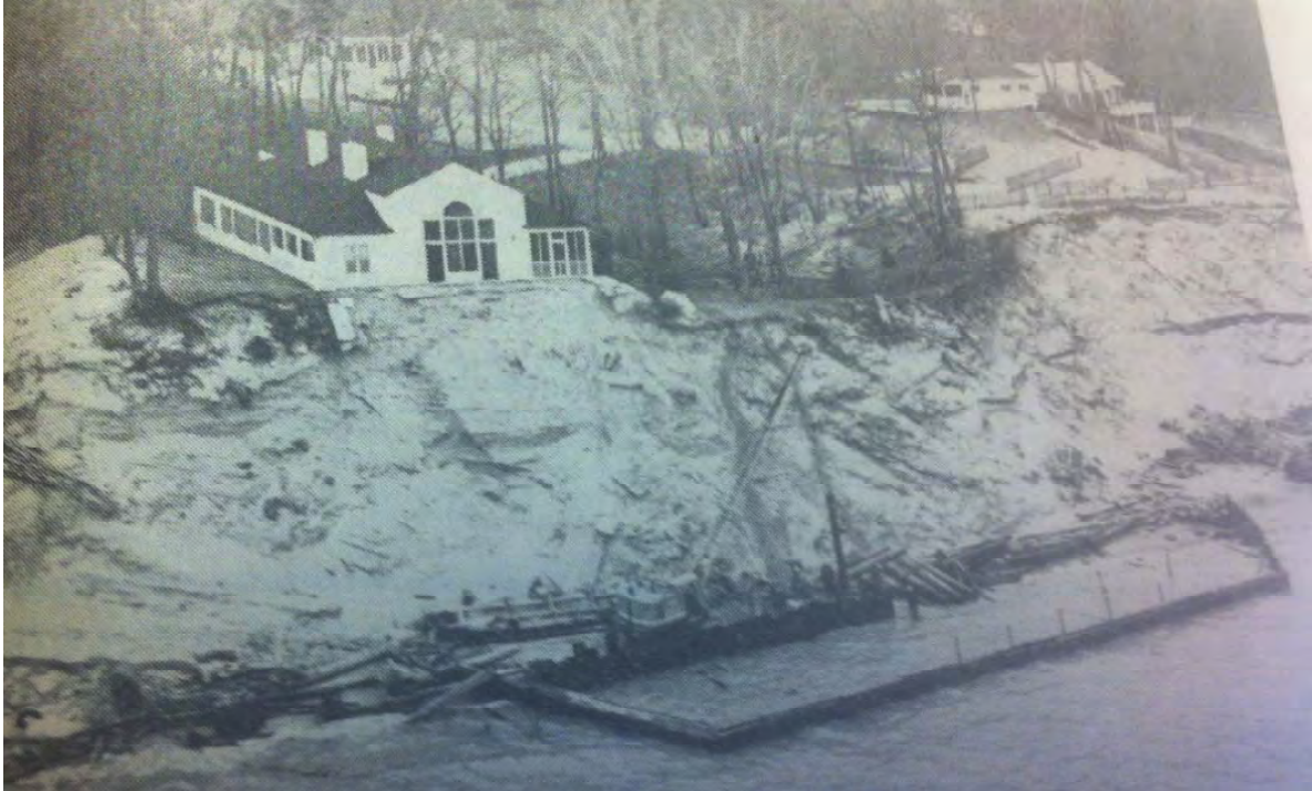
Figure 25: 1970s Herald Palladium photo of bluff erosion south of St. Joseph, MI
