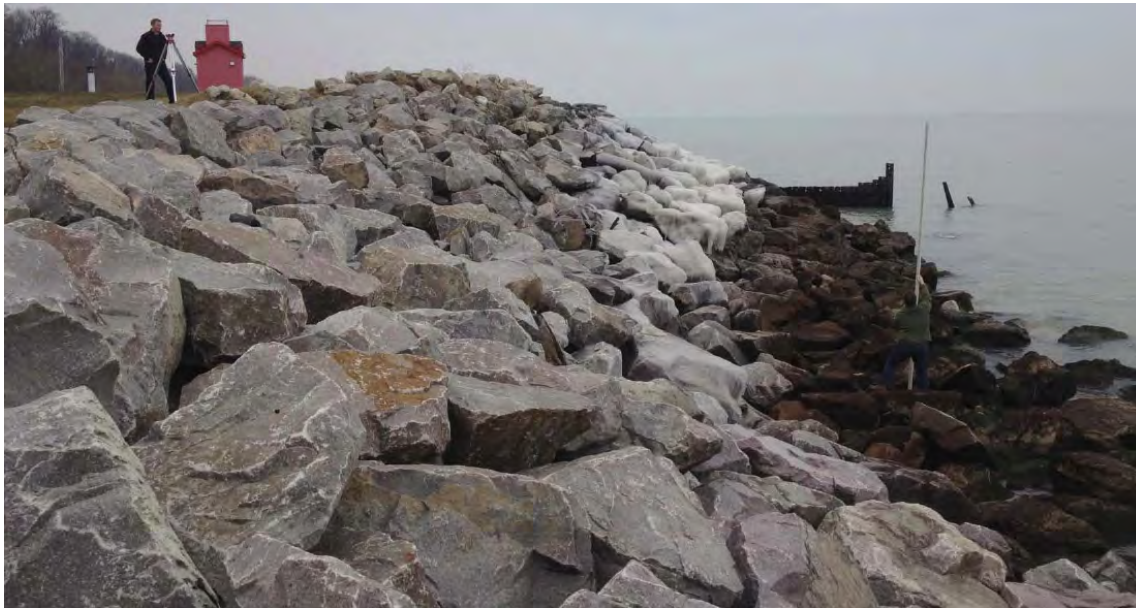
Figure 35: St. Joseph Water Plant Revetment, spring 2012
