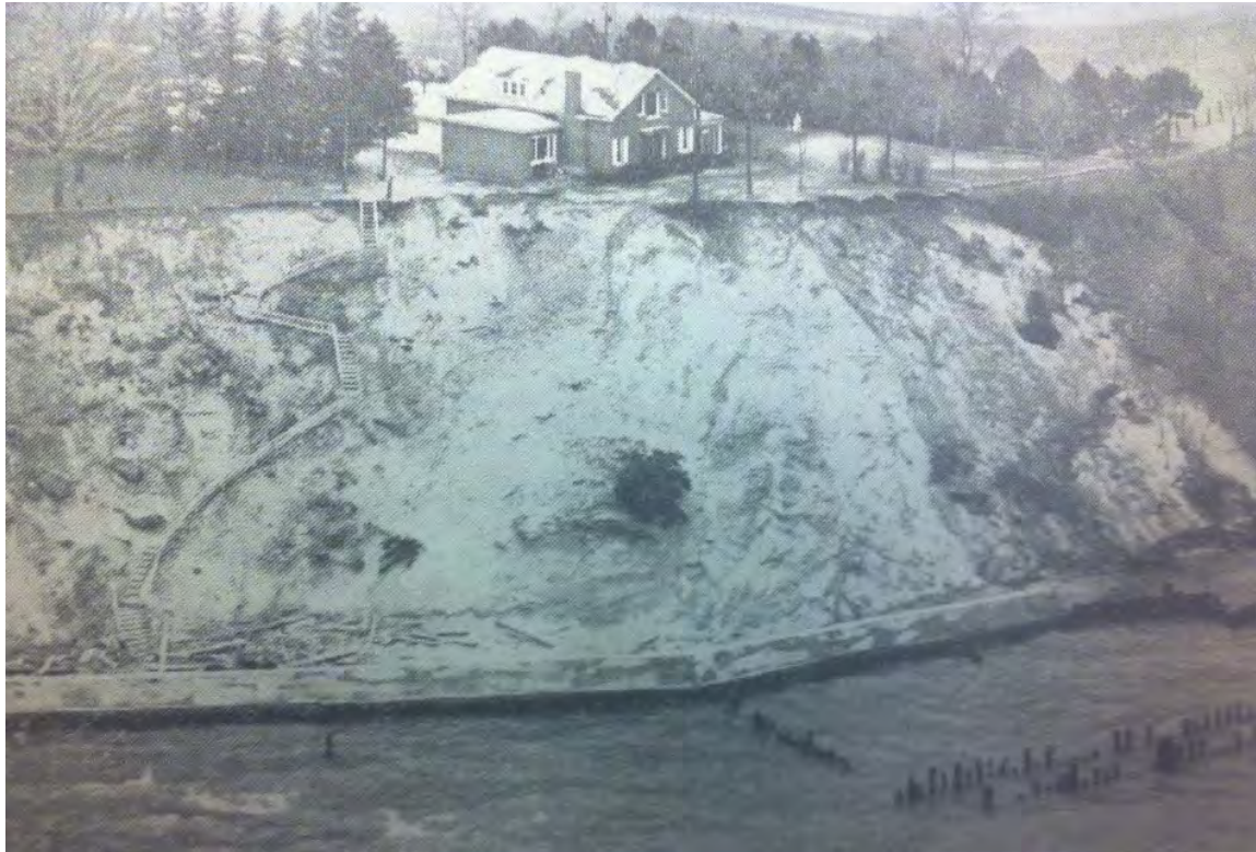
Figure 26: 1970s Herald Palladium photo of bluff erosion south of St. Joseph, MI
