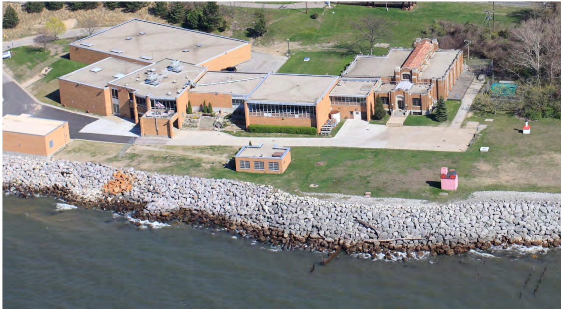
Figure 34: St. Joseph Water Plant Revetment Oblique Photo
