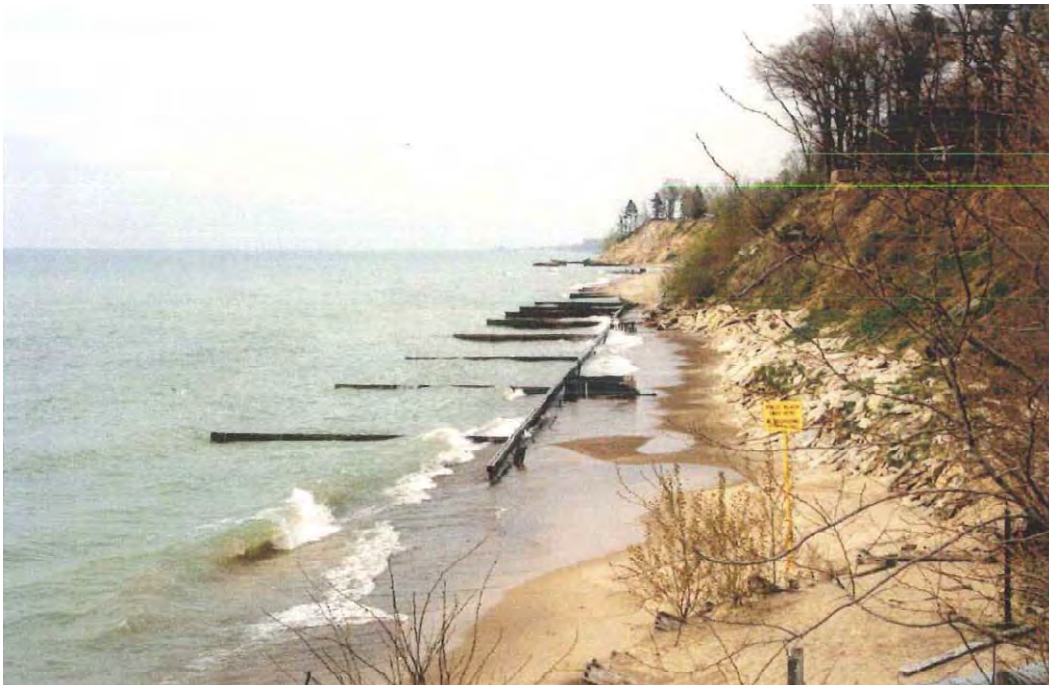
Figure 33: USACE CEM Photo, “A steel sheet-pile wall and groin field has been ineffective at protecting this section of cohesive shore along the Berrien County shore of Lake Michigan, south of the town of St. Joseph, April 1994.”
