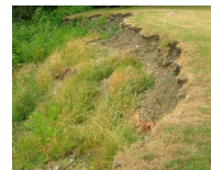
Example of Slumping Source: ODNR Office of Coastal Management
